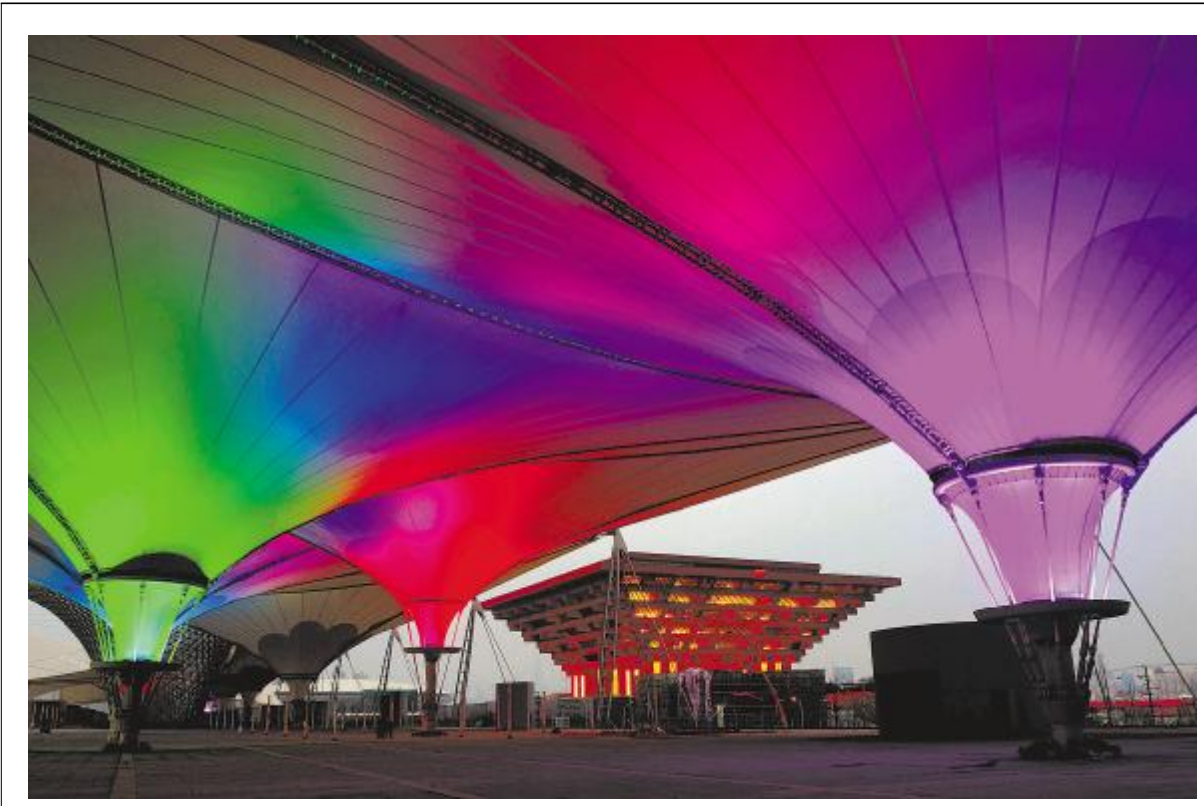
The LED energy-saving lights spotted on the brilliant cable-membrane structure of the axis during a trial illumination of Shanghai EXPO site on January 7.
