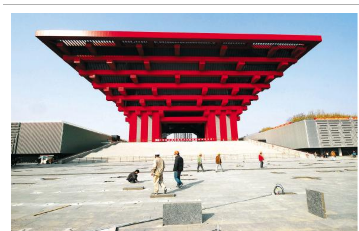
The January 21 marks the 100-day countdown to the opening ceremony of Shanghai Expo. Fitting-out works for the China Pavilion is now underway, one of the permanent buildings of Shanghai Expo.
